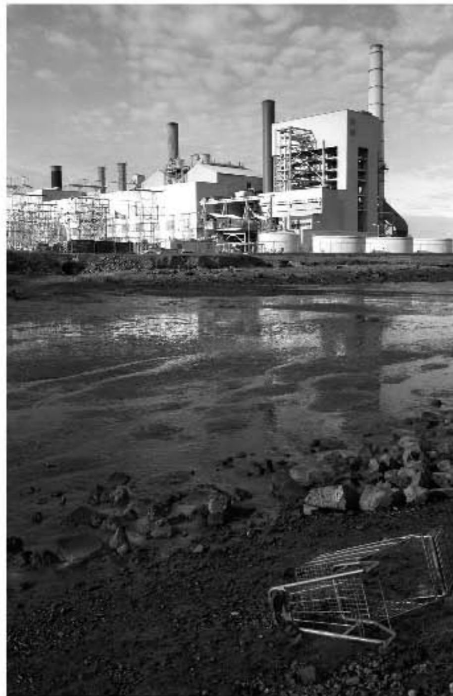
Hunters Point power station, San Francisco. 2006
